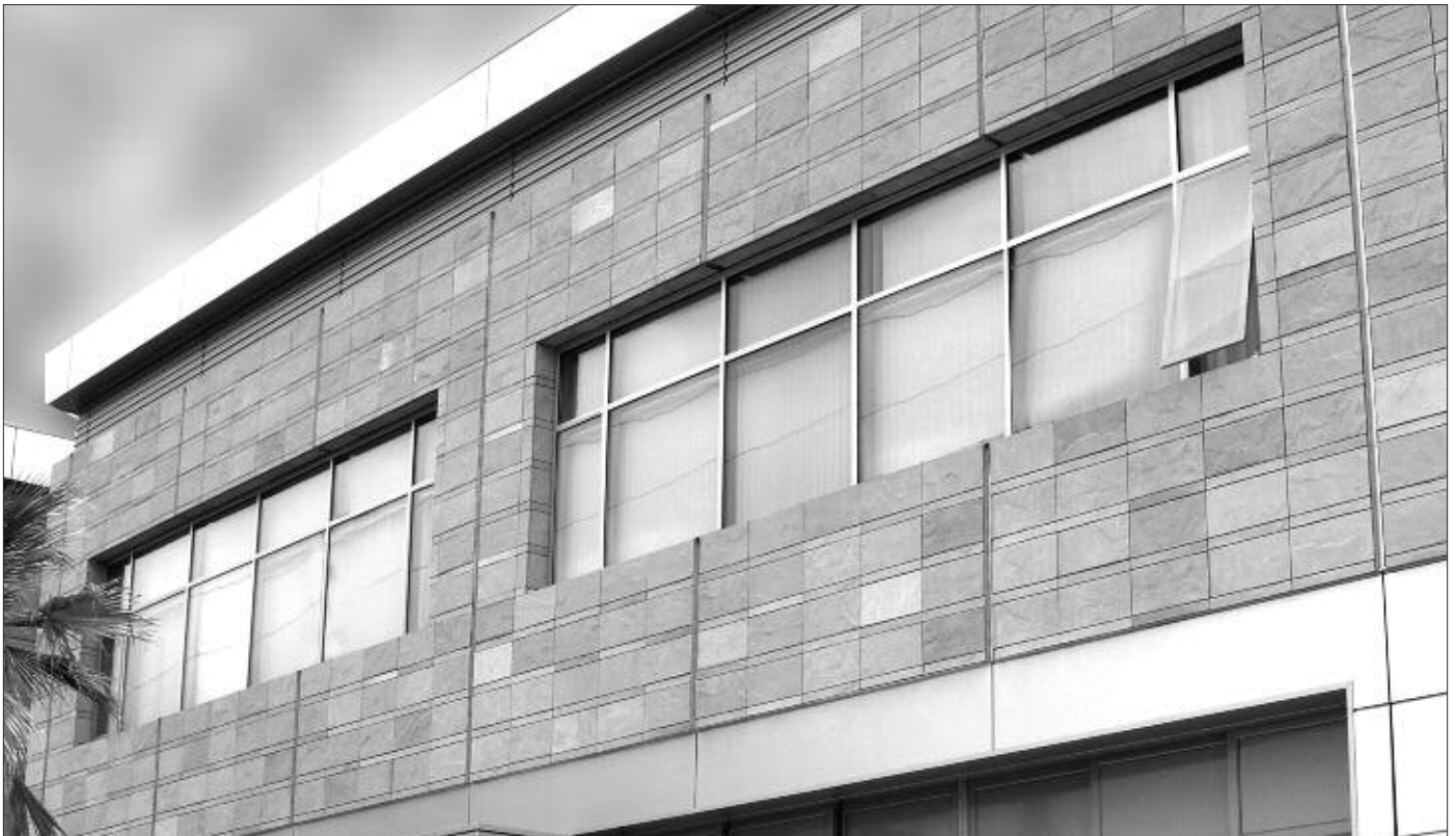
Project: Emergency Operations Command Center, Los Angeles, CA
