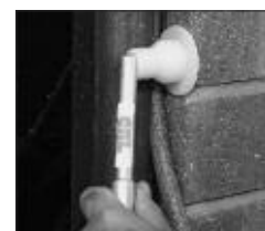
Part No. SBRR Roller Tool will not tear "skin" of Backer Rod.
