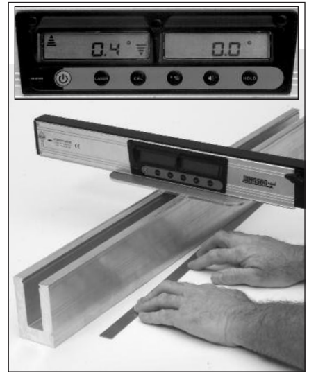
Use the "PAL" Tool to assure the Base Shoe is level at all points. When leveling the Base Shoe make sure you level the shoe within 0.4 degrees of the floor. Angular variation up to 0.4 degree is acceptable during this process.
