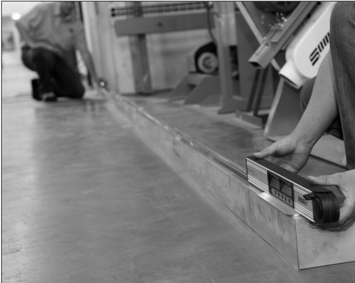
Align the "PAL" Tool with Windscreen Base Shoe and point toward the Laser Target set at opposite end.
