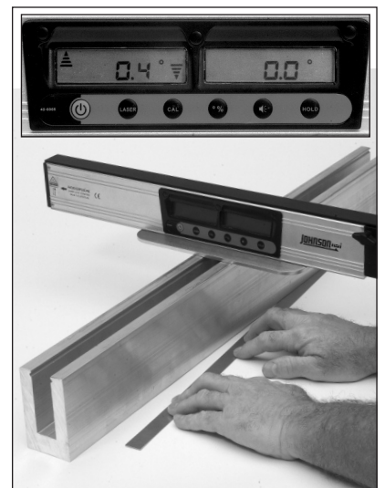
Use the "PAL" Tool to assure the Windscreen Base Shoe is level at all points. When leveling the Windscreen Base Shoe make sure you level the shoe within 0.4 degrees of the floor. Angular variation up to 0.4 degree is acceptable during this process.
