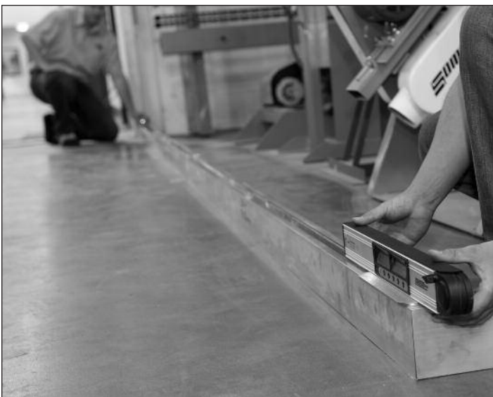
Align the "PAL" Tool with base shoe and point toward the Laser Target set at other end of Base Shoe.
