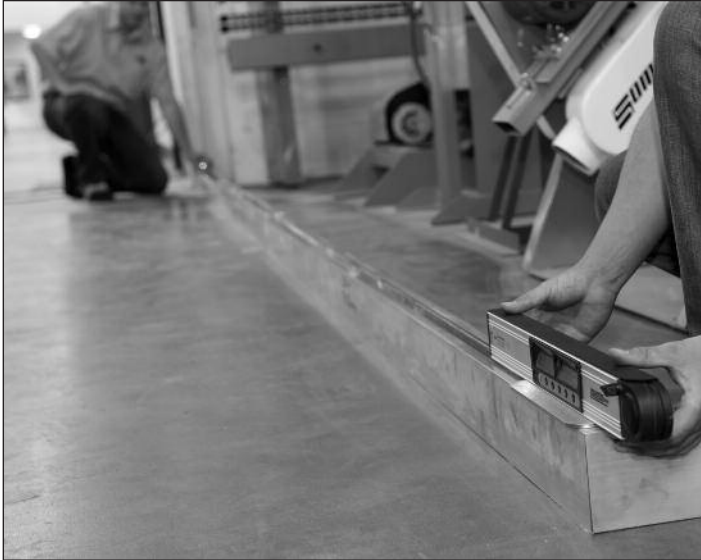
Align the "PAL" Tool with Base Shoe and point toward the Laser Target set at opposite end.
