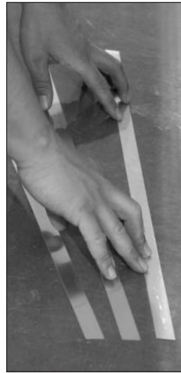
Slide Shim Strips under Base Shoe to fill gaps.
