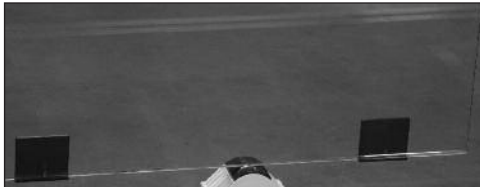
Make sure the TAPER-LOC™ spacing does not exceed 14" (356 mm) on center.
