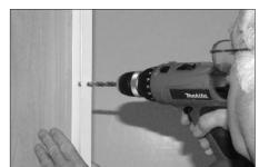
Diagram 13 - Prepping Side Jambs for Surface Mount Installations
