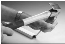
Diagram 8 - Crimping Weatherstrip Channel
