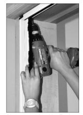
Diagram 10 - Attaching Top into Header
