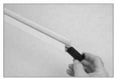
Diagram 6 - Installing Plastic Angle Brackets
