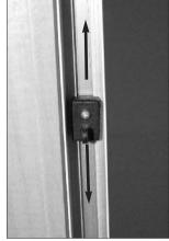
Diagram 12 - Adjusting Plastic Hook Latch
