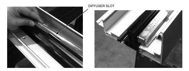
5. Silicone the diffuser to the divider riser along the exposed surface from end-to-end. Be careful not to block the breather holes with sealant.
